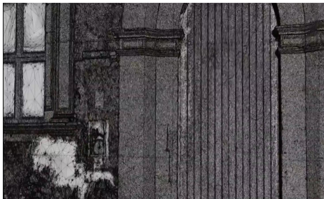
Laser scanning ( LiDAR )
